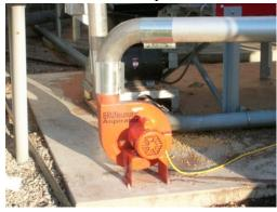
NOTE: The housing of the BRUNeumatic Aspirator may be turned in 90 degree segments, sometimes saving the installation of one elbow. See the end of this manual for instructions on how to do this.
